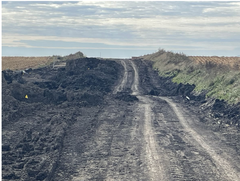
Facing south at MP 33.7, south of 165th Street; backfill repaired drain tile, subsoil grading, decompaction, ECD removal, and topsoil restoration
