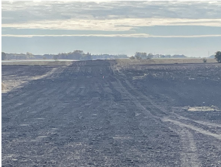
Facing south at MP 32.95, south of 154th Street; awaiting topsoil decompaction (discing)
