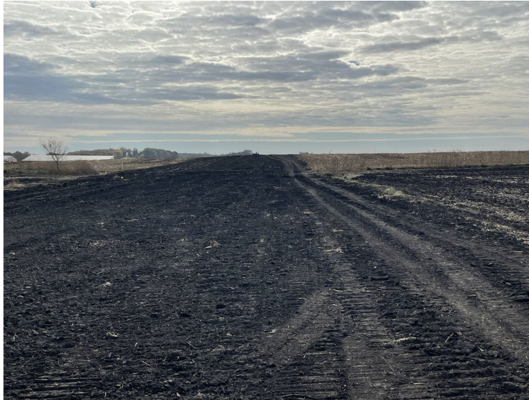
Facing south at MP 32.7, south of 154th Street; awaiting topsoil decompaction (discing)
