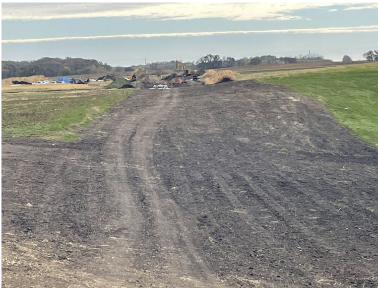
Facing south at MP 31.45, south of 140th Street; temporary workspace awaiting topsoil decompaction (discing), seeding (winter rye)/mulching/crimping
