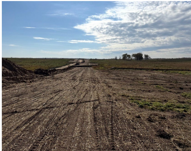
Facing south at 1.30, ROW restored up to a travel lane
