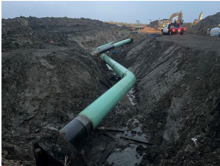
Facing north at MP 31.2, north of 135th Street (south tie-in location; temporary workspace with open trench awaiting drain tile repairs, backfill, subsoil grading, decompaction and topsoil restoration, E-line crossing under D-line
