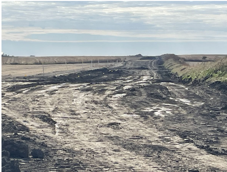
Facing south at MP 34.2, south of 165th Street; awaiting backfill repaired drain tile, subsoil grading/decompaction, topsoil restoration, ECD removal
