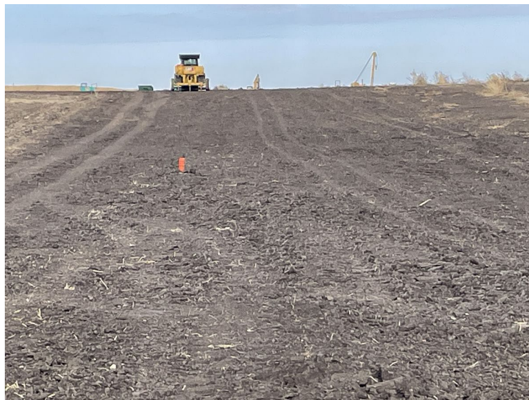
Facing north at MP 32.95, south of 154th Street; awaiting topsoil decompaction (discing)
