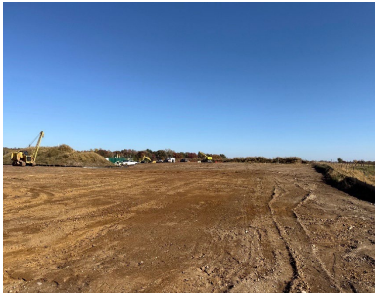
Facing north at MP 0.18, east side of the ROW (towards the Hugo station), awaiting topsoil restoration
