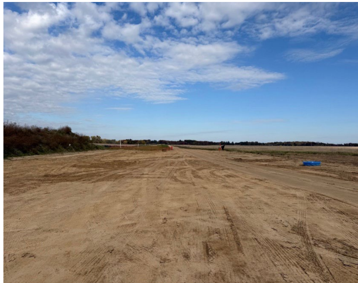
Facing east at MP 1.70, workspace awaiting restoration
