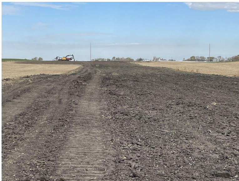
Facing north at MP 31.7, south of 140th Street temporary workspace awaiting topsoil decompaction (discing)
