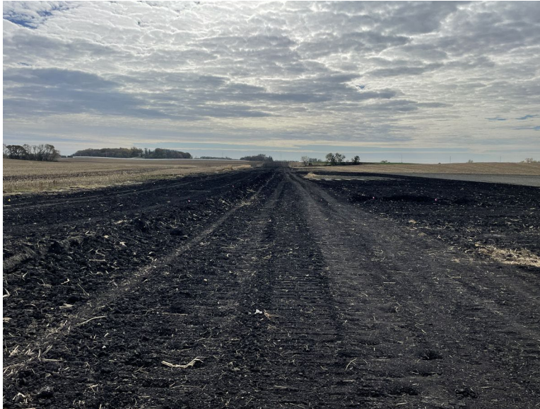
Facing south at MP 32.45, south of 154th Street; temporary workspace awaiting grading/decompaction (discing) topsoil
