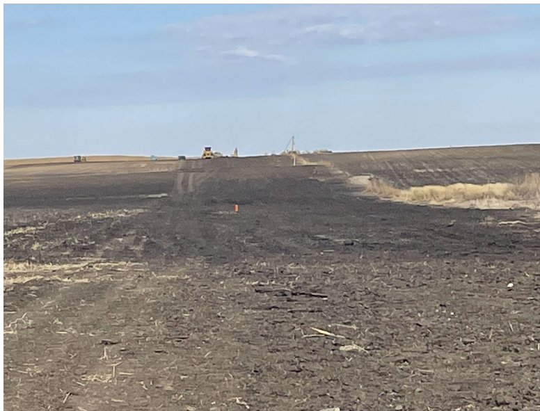
Facing north at MP 32.7, south of 154th Street; awaiting topsoil decompaction (discing)
