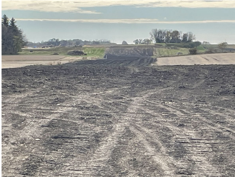
Facing south at MP 31.95, south of 140th Street; temporary workspace awaiting topsoil grading/decompaction (discing)
