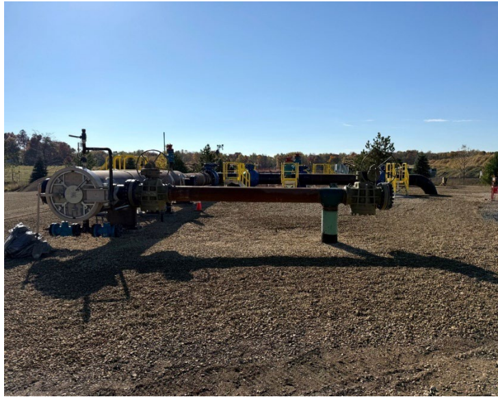
Facing south, view from the SW corner of the Hugo compressor station MP 0.1
