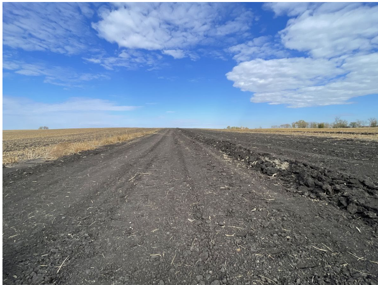
Facing north at MP 32.45, south of 154th Street; awaiting topsoil to grade/decompaction (discing)
