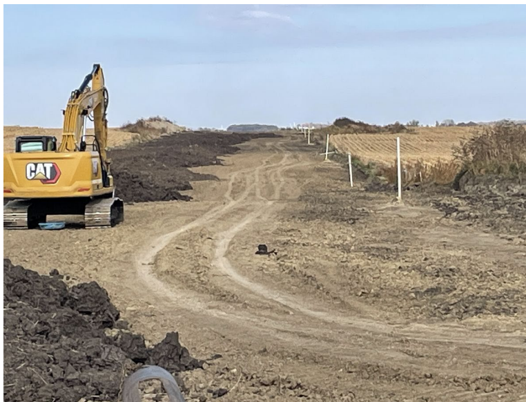
Facing north at MP 33.2, north of 154th Street; temporary workspace awaiting, removal of story poles, and topsoil restoration
