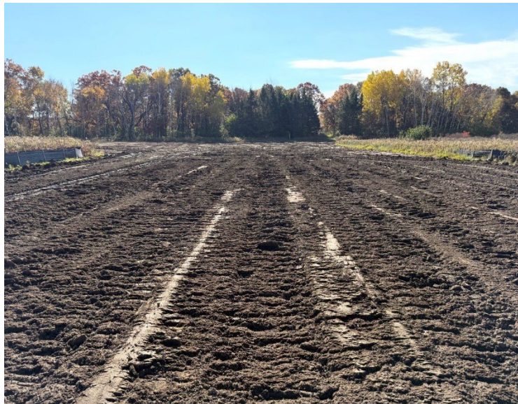
Facing south at MP 0.60, topsoil restored, awaiting final decompaction
