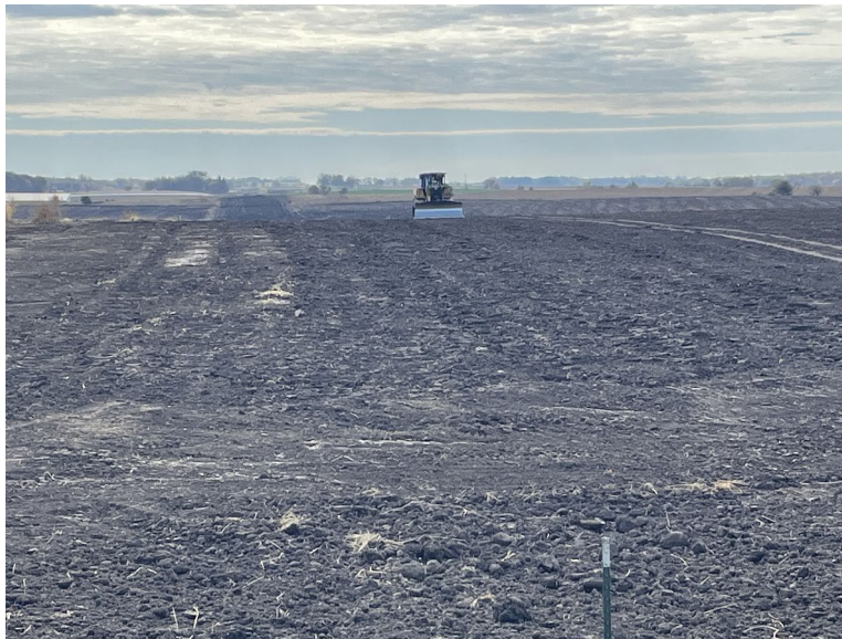
Facing south at MP 33.2, south of 154th Street, temporary workspace awaiting topsoil decompaction (discing)
