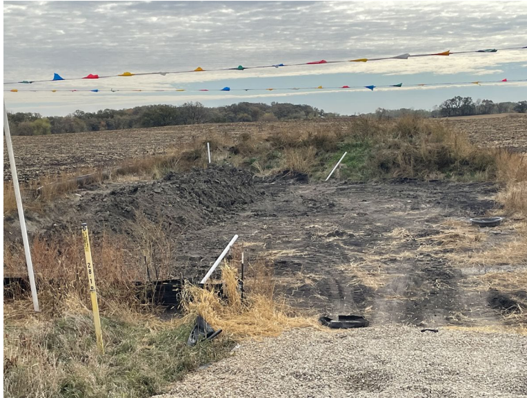
Facing south at MP 31.2, south of 135th Street at the discontinued line stop location; awaiting drain tile repair, backfill, decompaction, ECD removal, and topsoil restoration
