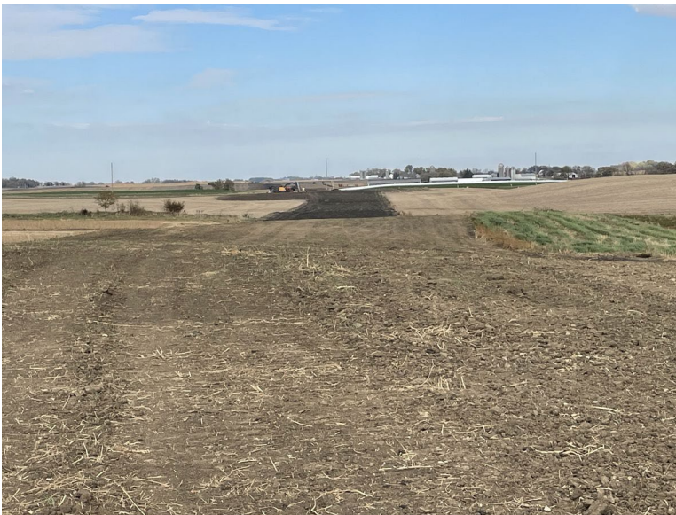
Facing north at MP 31.45, south of 140th Street; temporary workspace awaiting topsoil decompaction (discing), and temporary seeding (winter rye) mulching/crimping
