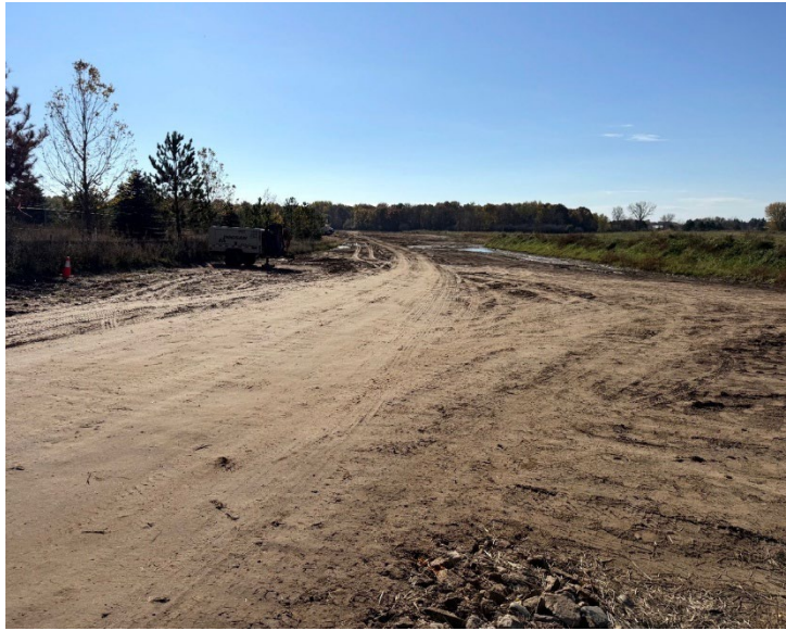
Facing south near MP 0.1, ROW from the access road on the west side of the Hugo Compressor Station
