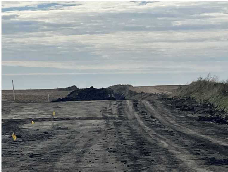
Facing south at MP 33.95, south of 165th subsoil brought to grade awaiting drain tile backfill decompaction, topsoil restoration, and ECD removal
