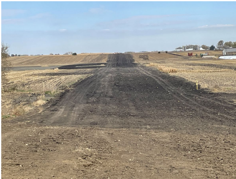
Facing north at MP 32.2, north of 140th Street; awaiting topsoil decompaction (discing)
