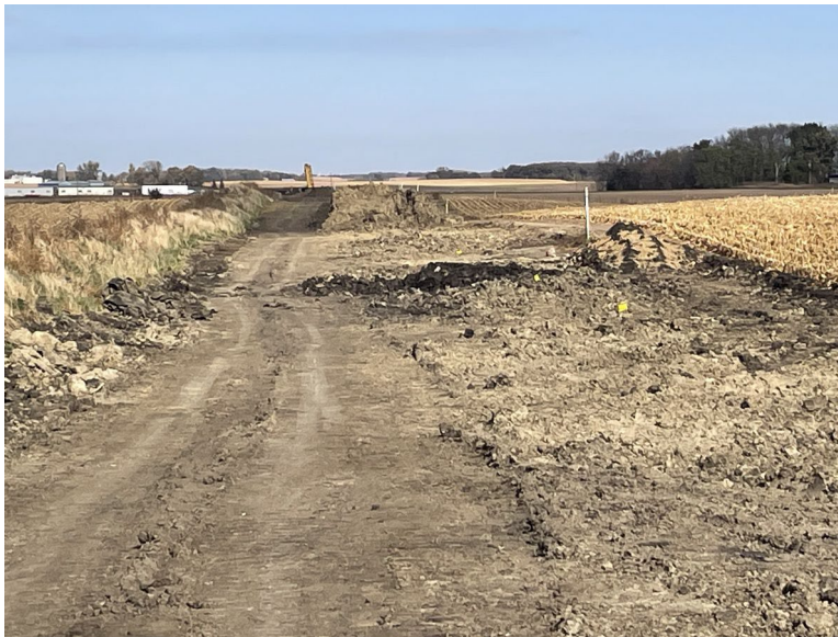
Facing north at MP 33.7, south of 165th Street, subsoil grading/decompaction, backfilling repaired drain tile, ECD removal, and topsoil restoration
