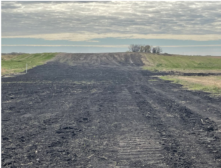
Facing south at MP 31.7, south of 140th Street; temporary workspace awaiting topsoil decompaction (discing)
