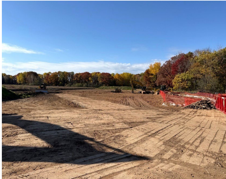
Facing west at MP 0.55, clean up in progress
