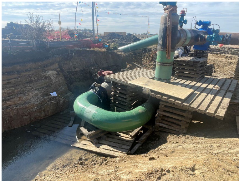
Facing west at MP 34.2, north of 165th Street; tie-in complete awaiting concrete support installation, sandblasting/coating, backfill, subsoil grading, and topsoil restoration
