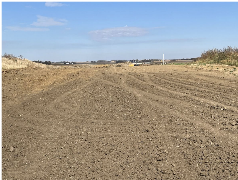
Facing north at MP 33.45, south of 165th Street; temporary workspace awaiting ECD removal, and topsoil restoration
