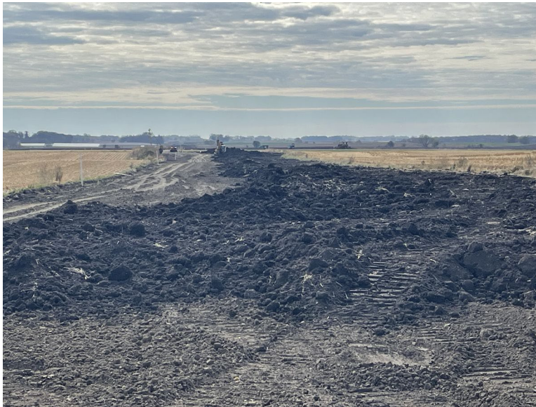
Facing south at MP 33.45, south of 165th Street; temporary workspace awaiting topsoil restoration
