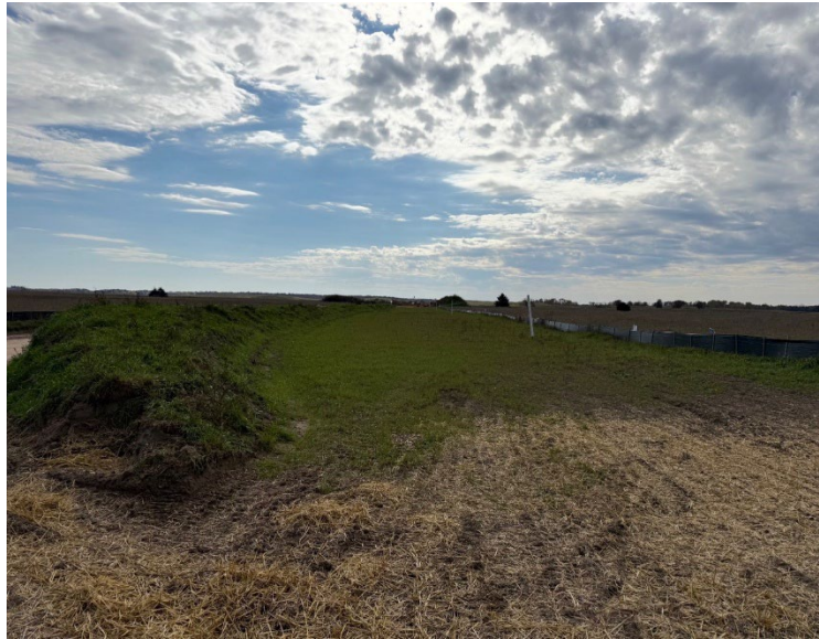
Facing south at MP 1.55, ROW restored up to a travel lane showing temporary vegetation
