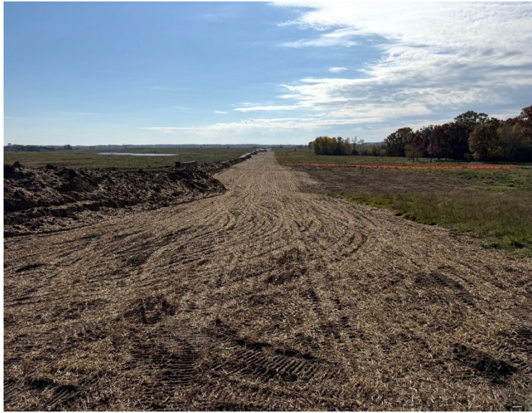
Facing south at MP 1.0, ROW restored up to a travel lane
