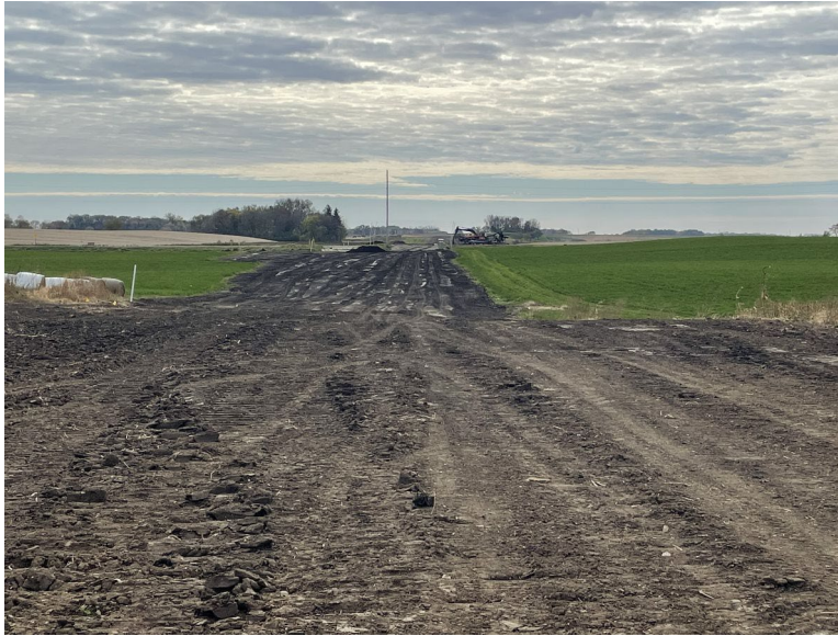
Facing south at MP 32.2, north of 140th Street; awaiting topsoil to grade/decompaction (discing), seeding (winter rye), and mulching/crimping
