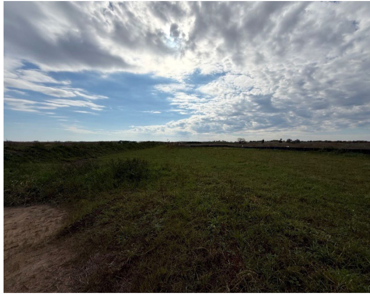
Facing south at MP 1.75, ROW restored up to a travel lane
