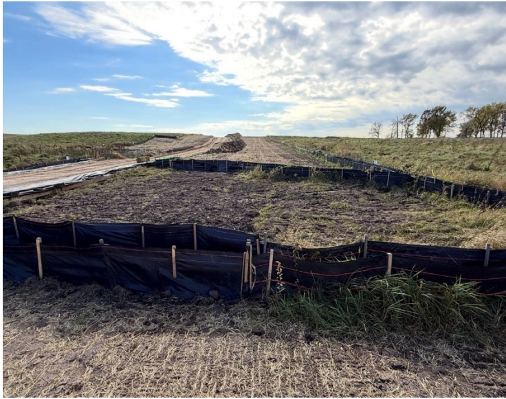
Facing south at MP 1.38, wetland FRM-W12 restored
