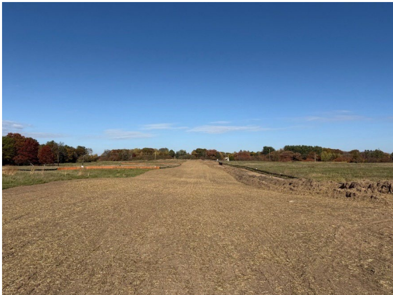
Facing north at MP 1.25, ROW restored up to a travel lane
