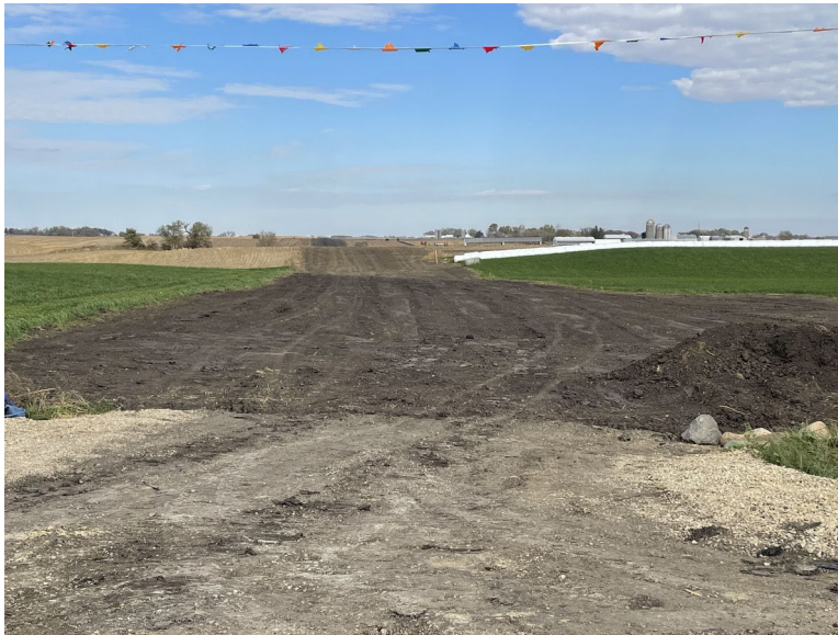
Facing north at MP 31.95, north of 140th Street; temporary workspace awaiting topsoil decompaction (discing), seeding (winter rye), and mulching/crimping
