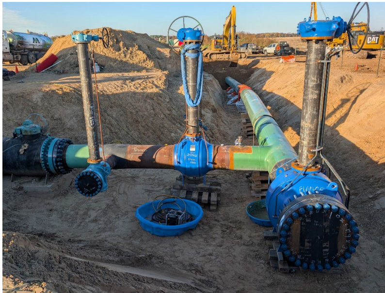
Facing north at MP 1.9, bell hole with the Farmington Tie Over Valve Setting final tie-in activities, completed October 27, 2025
