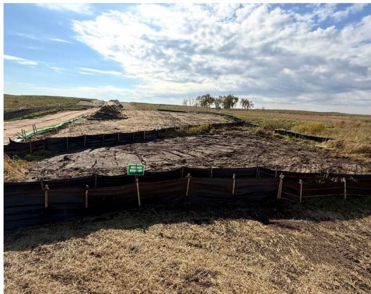
Facing south at MP 1.35, wetland FRM-W13 restored
