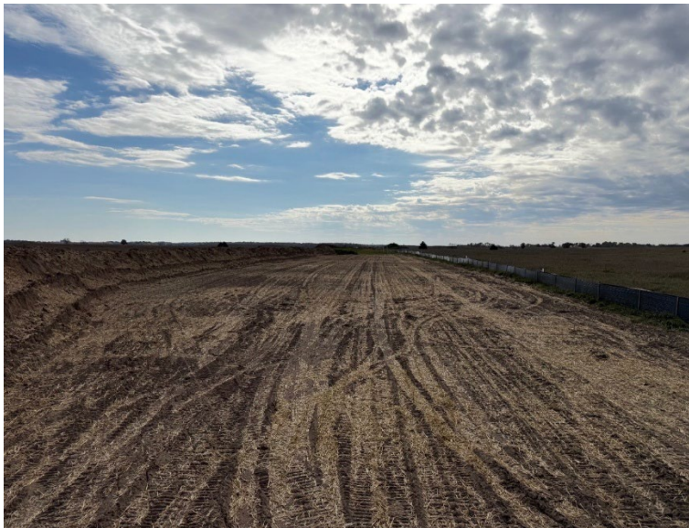
Facing south at MP 1.45, ROW restored up to a travel lane
