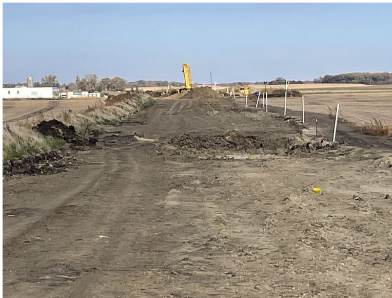
Facing north at MP 33.95, south of 165th Street; awaiting backfill repaired drain tile, subsoil grading/decompaction, ECD removal, and topsoil restoration
